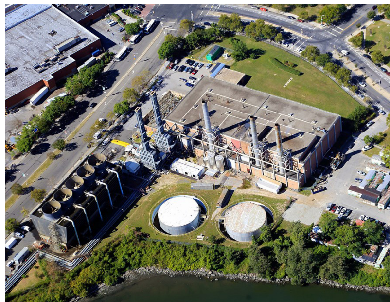
Riverbay Cogeneration Facility*
